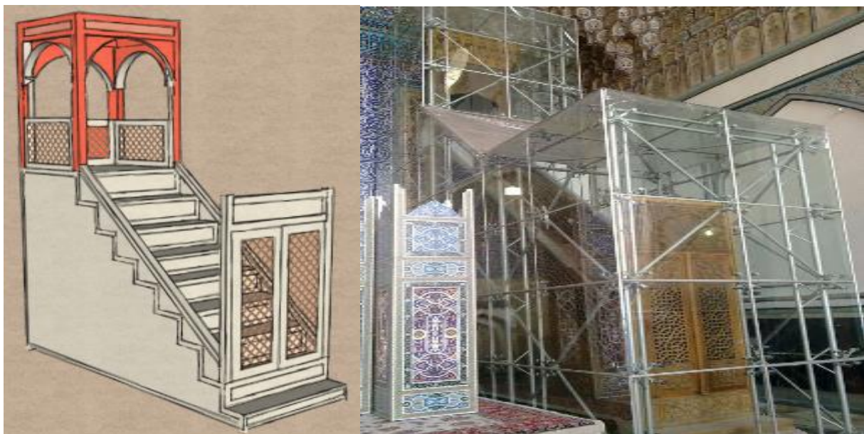
Fig. 10. the installation of chamber room in Goharshad Jami Mosque (Author).
