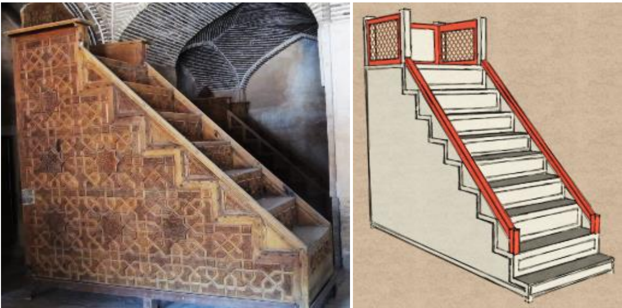
Fig. 6. the Installation of handrails in Jami Mosque of Isfahan (Author).
