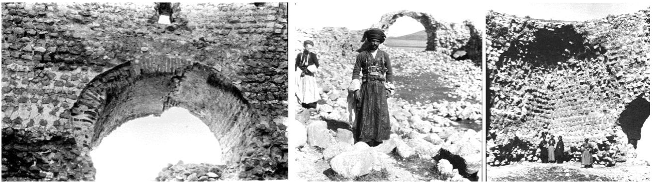
Fig. 6. Brick arch, the eastern gateway, part of the dome (Bell, 1914).
